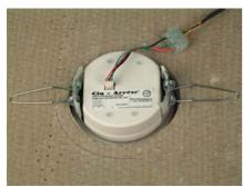
The CSA-REFUV is installed into a suspended ceiling tile or other false ceiling by cutting a 110mm / 4  $^{1}$ /41 inch  $\Phi$  hole in the ceiling tile or lining.
